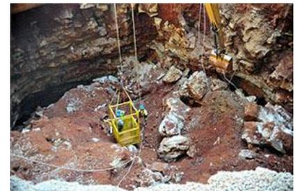
Dr. Jason Polk with WKU shared that the void discovered beneath the Skydome extended in two directions – one leading from the Skydome towards the Museum's truck parking lot, and the other leading from the Skydome towards the pond. Both cave areas start approximately 50 feet underground. According to Dr. Polk, "You don't typically have sinkholes without caves or voids of some type below them, so this finding was not surprising."
